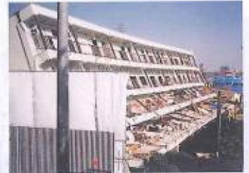
Collapsed apartment building near the epicenter at Kobe, Japan (Photographed on Feb. 11, 1995)
