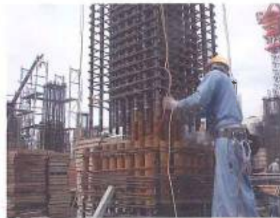
Slim Sleeve for connecting rebar cage
