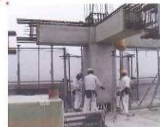
Erecting precast column
