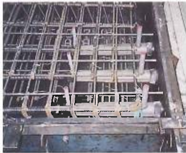
Precast wall before pouring concrete
