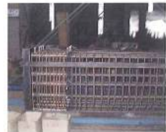
Assembling rebar cage for precast column
