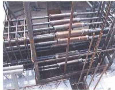
Slim Sleeve for connecting beam rebar
