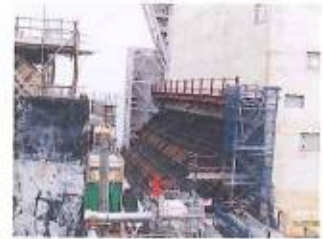
Akashi Channel Bridge, Anchorage
