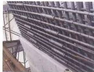
Bridge Pier Reinforcement
